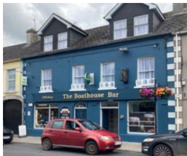
Streetscape Enhancement Scheme 2023-24 in Portumna
